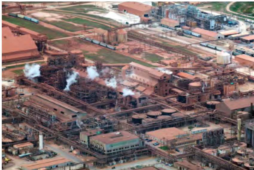
Figure 25.1: An aluminium production plant
